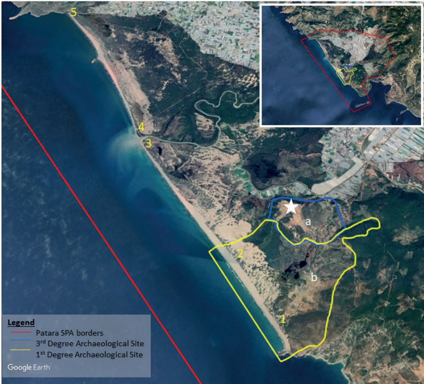
Fig. 1. Patara SPA GoogleEarth Map. White star: construction site of summer house village. a) new second road connecting villas and Gelemis village. b) archaeological site fee collection point with daytime vehicle barrier. Nos 1-5 are entry points: 1: Patara main beach entry point, snack bar & beach furniture; 2: entry point via sand dunes, connecting beach with summer house village; 3: Çayağzı beach entry point & illegal beach bar (est. 2014, closed in 2015); 4: Letoon beach entry point and abandoned SPA information kiosk; 5: Özden beach entry point, bar, camping site, 4x4 rentals (Özden river outlet). Esen river outlet lies between Nos 3-4.
